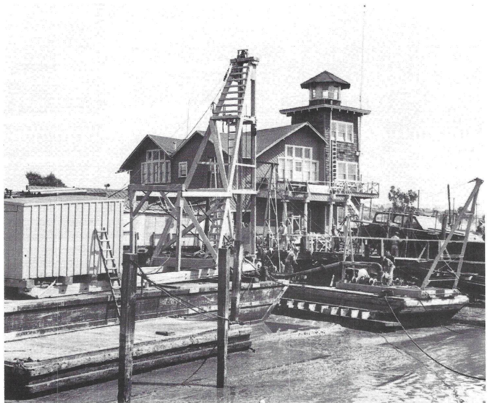
The pile drive (left) and club-member-built dredge were used to construct the present harbor. Photograph circa 1949-50.
